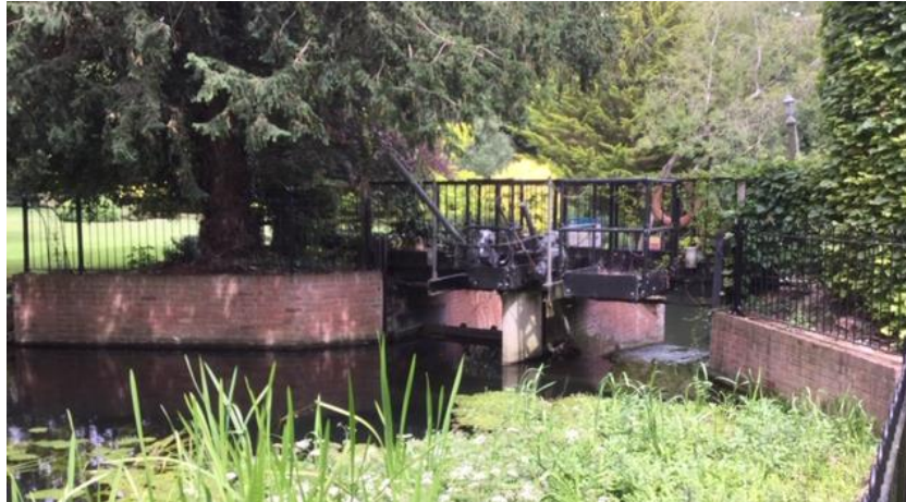
Image: Gressenhall Sluices, showing the two tilting gates.
